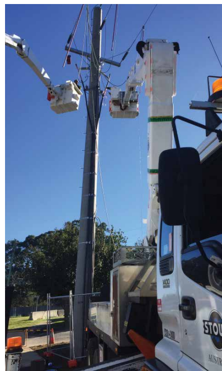
Above: Utility power pole replacement.
