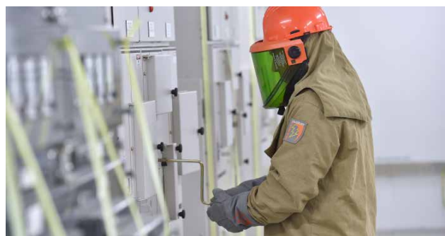
Above: High Voltage switching with 40Cal Arc Rated clothing.
