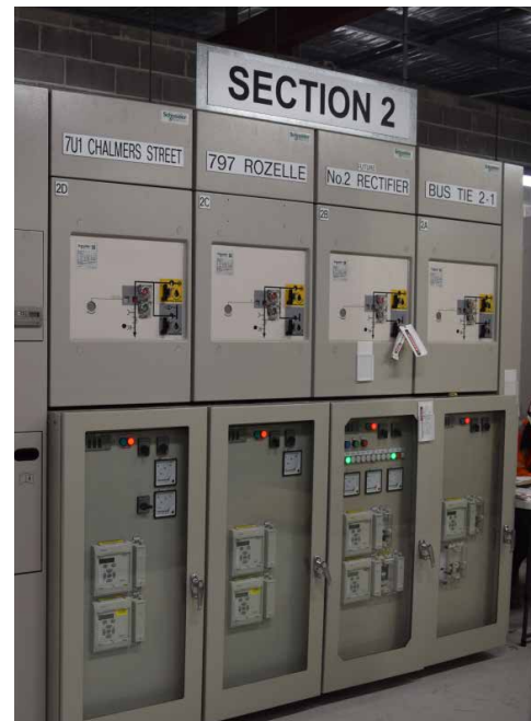
33kV switchboard at Lee Street traction substation, Sydney.
