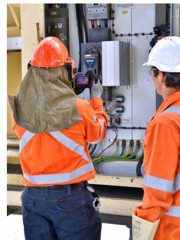
Top: Setting up for switchboard maintenance.
